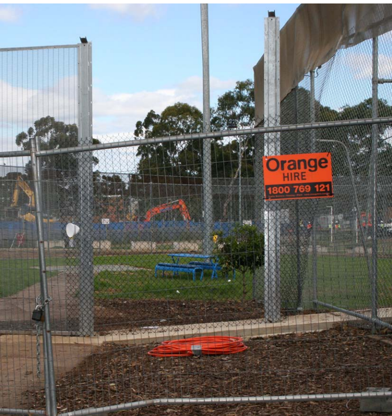
Construction works, Villawood Immigration Detention Centre.
