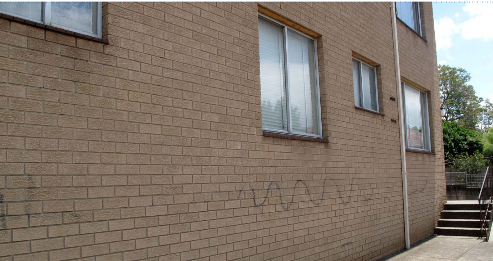
External view, flat occupied by family in community detention.
