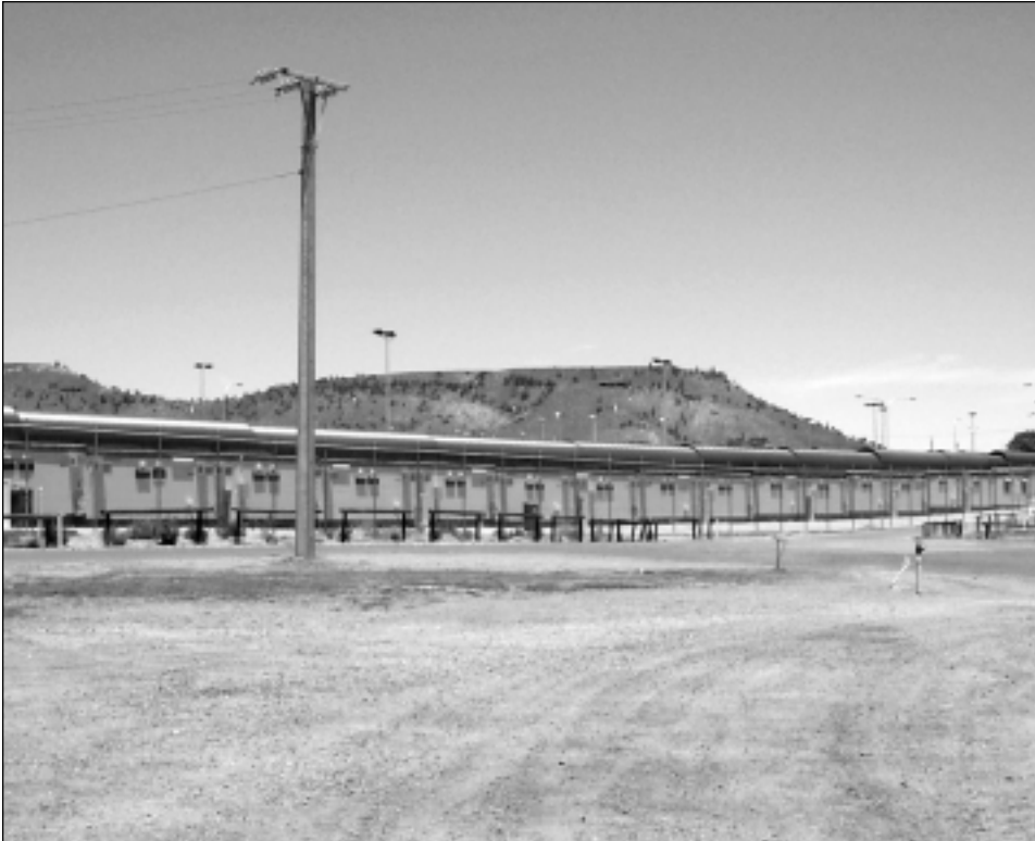
Exterior view of Baxter Immigration Detention Facility, December 2002.
